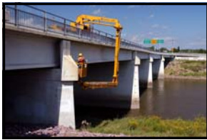
Steel bridge inventory
