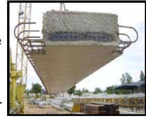
Precast section used in Pourtre Dalle System
